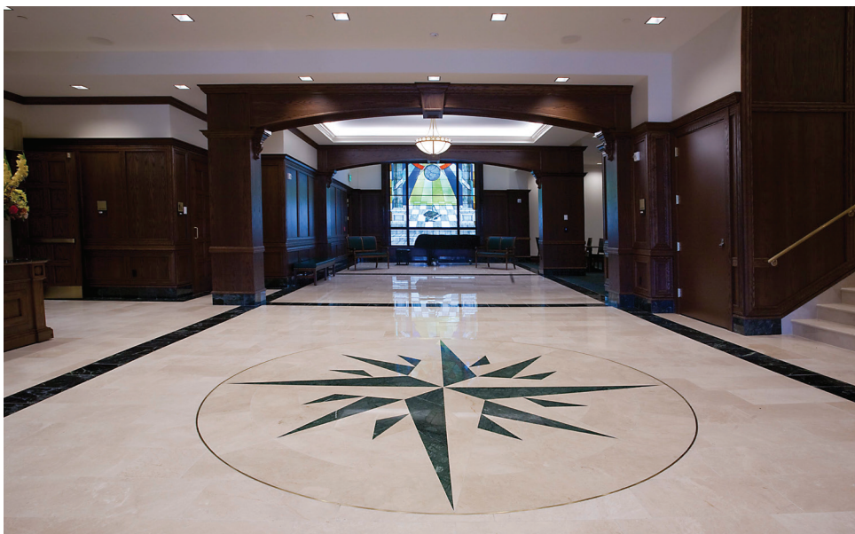
Above and below: To cap off and accent the beauty of the lobby, WTG installed a custom-made waterjet cut star emblem, utilizing the same materials and surrounded the star with a brass-circle. Credit: WTG Terrazzo
