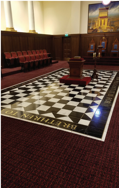
Above and below: The lodge area was installed with a 12"x12" Petra Slate Polished Nero and a 12"x12" Back Bay Marble Polished Bianco Venatino in a checkerboard pattern. The design consisted of three borders of the same material in a 45-degree triangle border pattern and a solid black pattern with custom waterjet-cut marble and brass lettering. The final border utilized the Polished Bianco in a 2-in. cut. Credit: WTG Terrazzo
