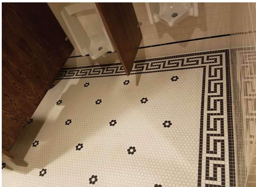
Hex Daltile Keystone daisy pattern on the main restroom floor. Credit: WTG Terrazzo
