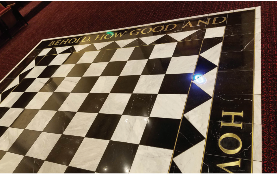
Above and below: The lodge area was installed with a 12"x12" Petra Slate Polished Nero and a 12"x12" Back Bay Marble Polished Bianco Venatino in a checkerboard pattern. The design consisted of three borders of the same material in a 45-degree triangle border pattern and a solid black pattern with custom waterjet-cut marble and brass lettering. The final border utilized the Polished Bianco in a 2-in. cut. Credit: WTG Terrazzo
