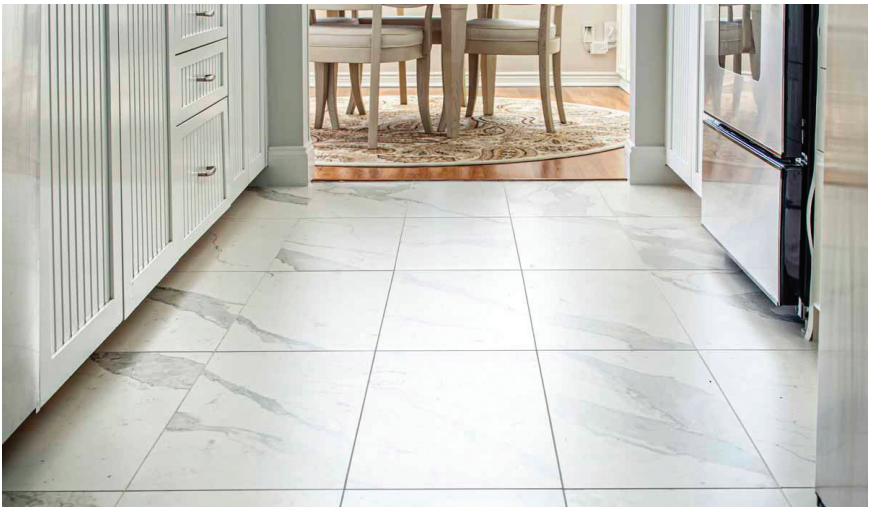
Clearwater Beach Condominium Kitchen Remodel - Clearwater, FL. As new owners of a beautiful beachfront condominium on the 11th floor, the family wanted to update the kitchen, including the floor and countertop. To ease the demo timeline, the team chose Crossville's porcelain tile panels for the kitchen floor in an easy, tile-over-tile installation. Credit: Crossville Inc.
