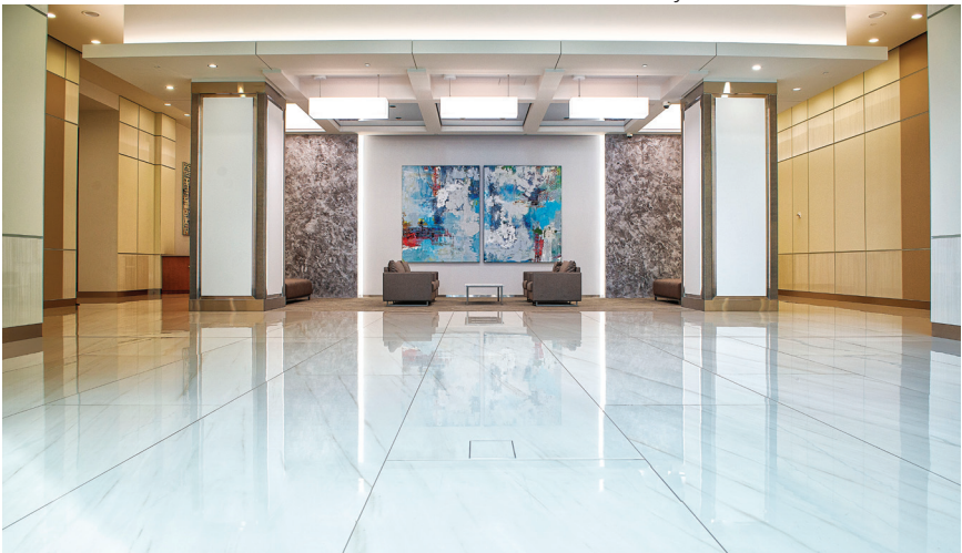
Bank of America Plaza at Las Olas City Centre - Fort Lauderdale, FL. Searching for a product that would be large-scale and could be installed over the existing floor, the design team found that Crossville's gauged porcelain tile panels in Cava provided a stylish solution to an upscale office renovation. Credit: Crossville Inc.
