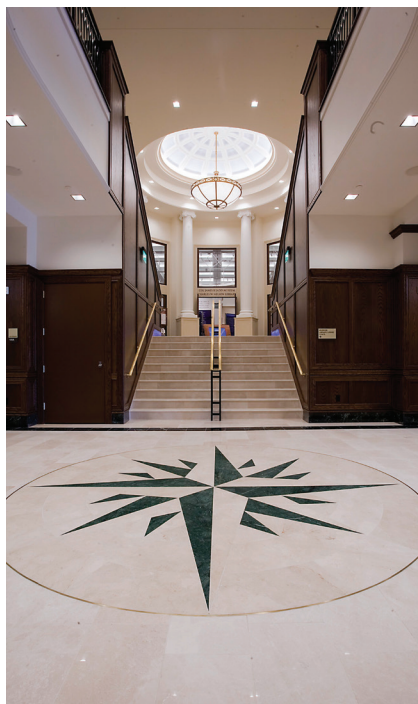
Above and below: To cap off and accent the beauty of the lobby, WTG installed a custom-made waterjet cut star emblem, utilizing the same materials and surrounded the star with a brass-circle. Credit: WTG Terrazzo
